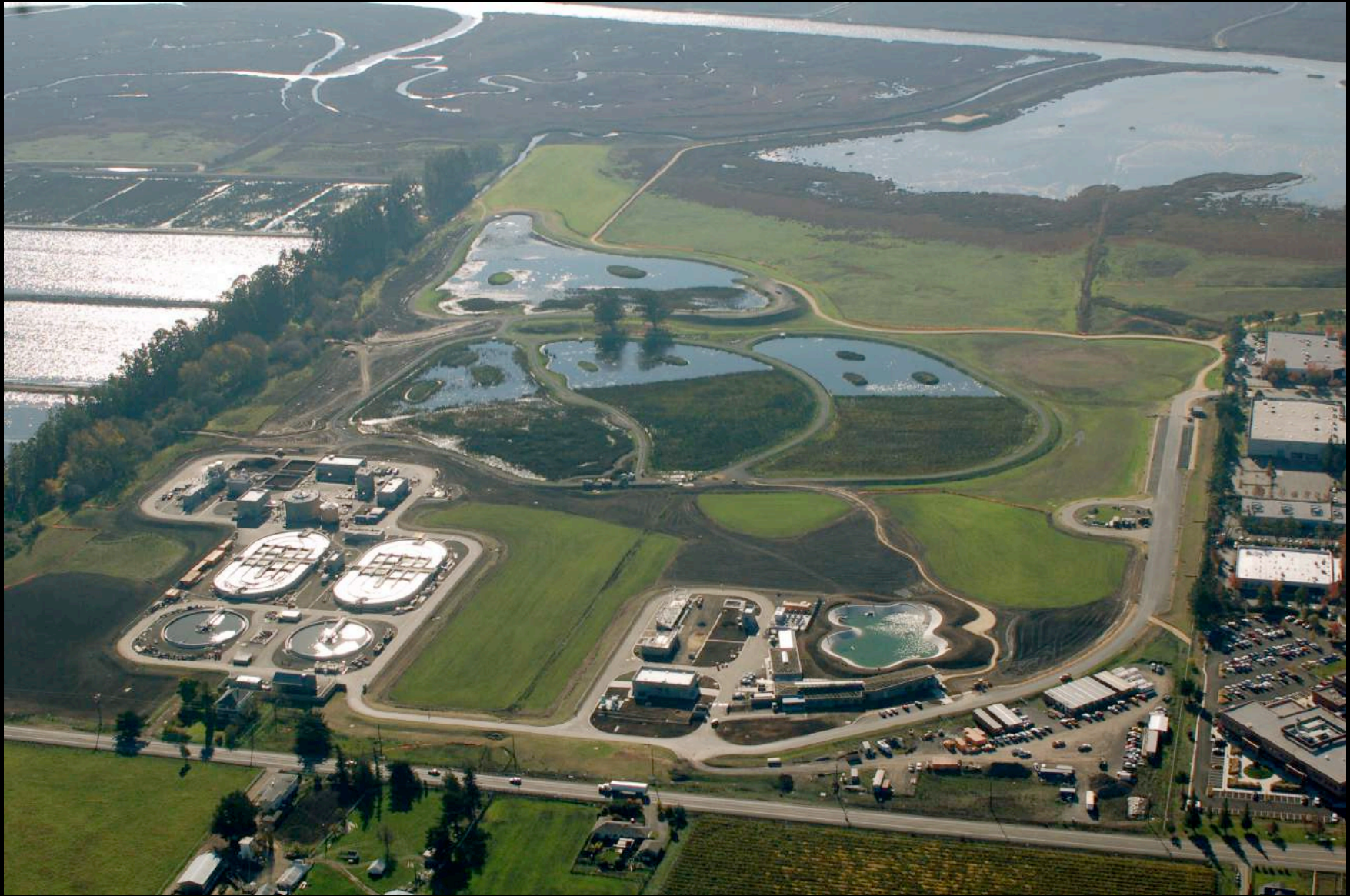
Patricia Johanson Ellis Creek Water Recycling Facility, Petaluma, CA
